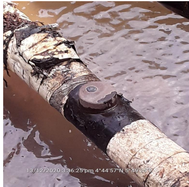
Fig D: Incident Facility during repair
